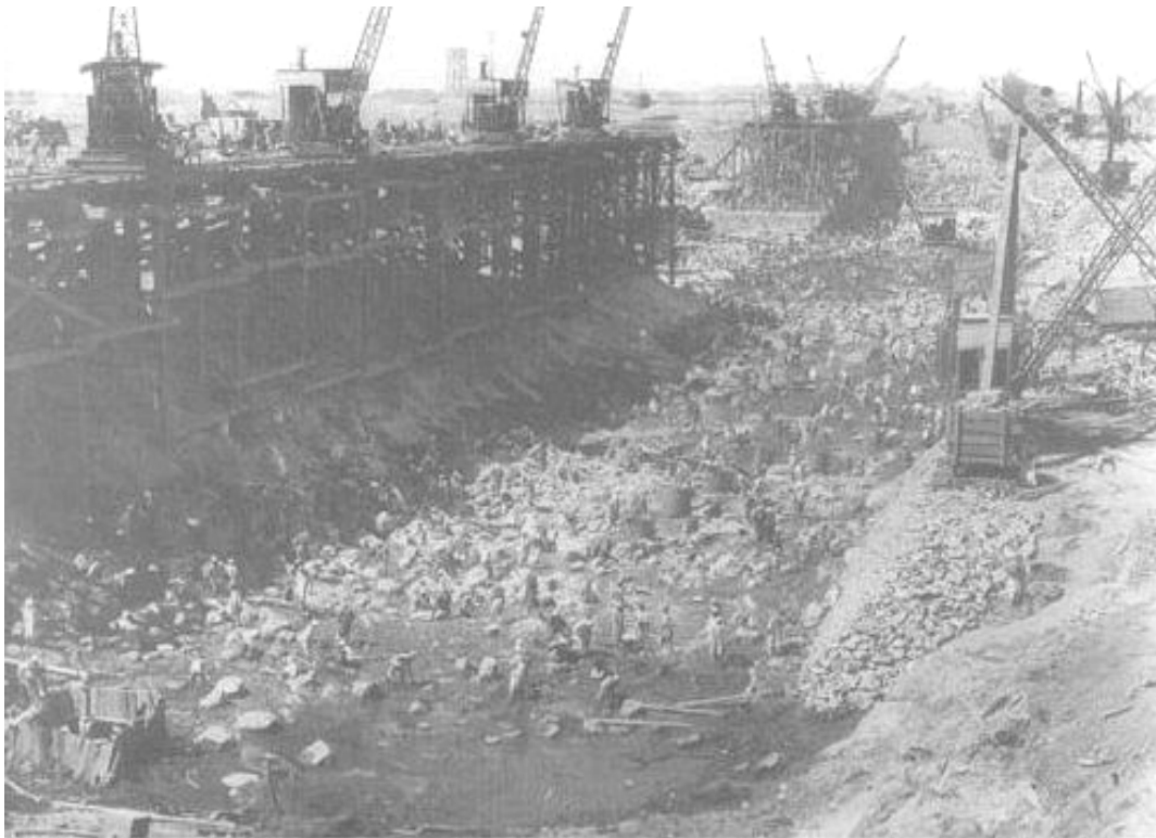
53 The Sennar Dam under construction, c. 1922. The project employed a combination of the newest technology and, in its use of labour, what a critic called 'Pharaonic methods'. PARKER COLLECTION, PHOTOGRAPHER UNKNOWN
