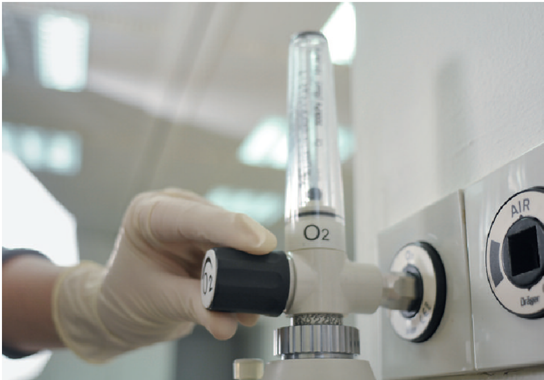
Fig(2-3) Theconventialflowmeter
