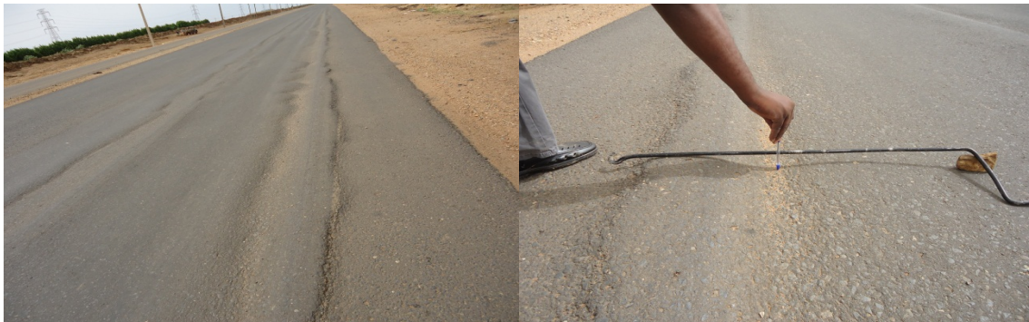
Figure 1.2: Rutting in Wheel Pass in Khartoum Ring Road
