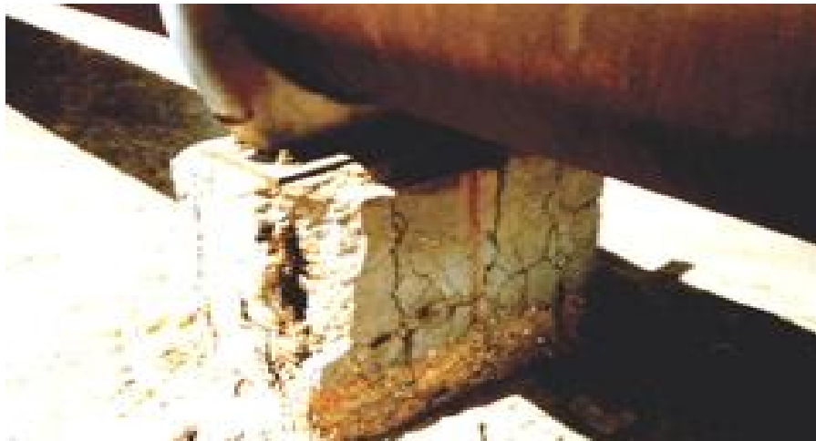
Fig. [2.1]: Sulphate attack on pipe pedestal.
