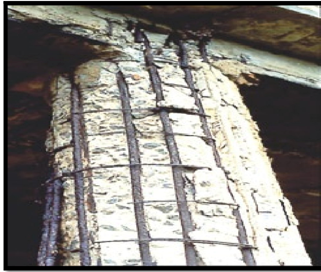
Fig. [2.2]: Poor Concreting in column.
