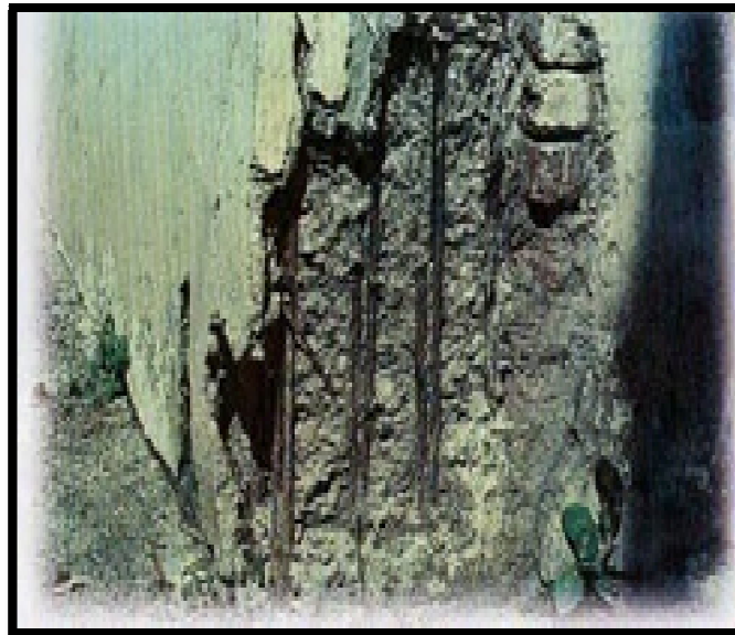
Fig. [2.3]: Poor quality of concrete in cover and ingress of moisture.
