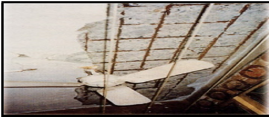
Fig. [2.4]: Less cover in slab bottom and cold joint.
