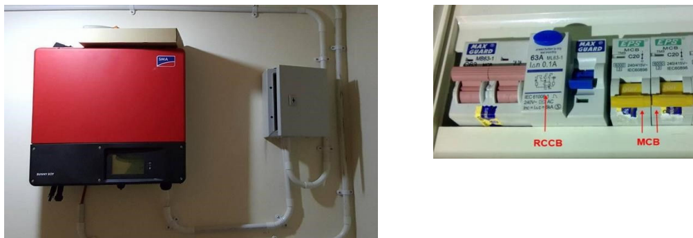
Figure 3-4: (a)The Connection of CB's With Inverter, (b) The Connection Between RCCB and MCB].
