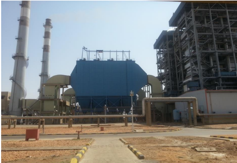
Figure A.1: Garri 4 power plant
