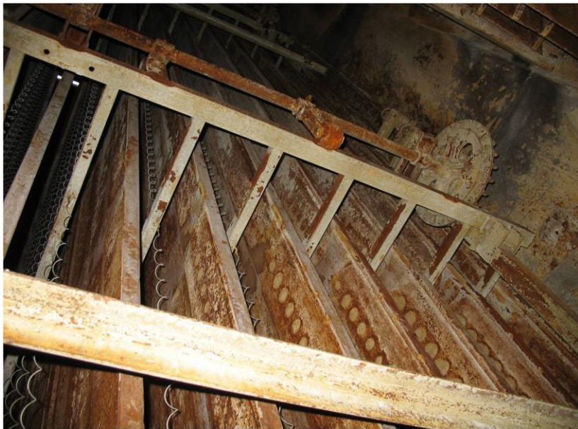
Figure A.4: Rapping mechanism
