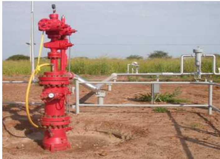
Figure C.1: Crude Oil Production Well [4].
