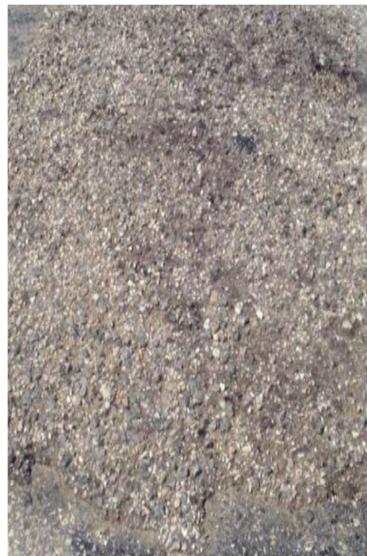
Figure 3.36 Medium Severity Raveling
