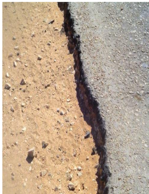
Fig. 3.23: Medium Severity Lane/Shoulder Drop-off
