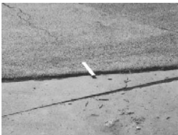
Figure 3.44 Low Severity shoving
