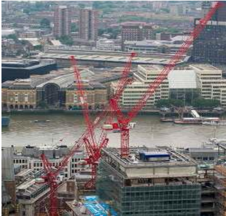
Figure 2.2: Luffing jibs.
