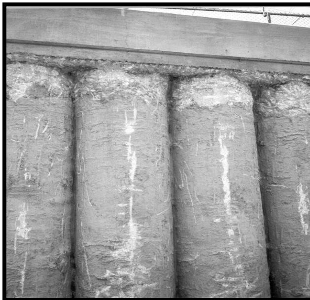
Figure 4-18 Tangent Pile Walls
