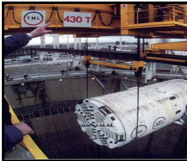
Figure 4-19 Lower Down TBM Machine
