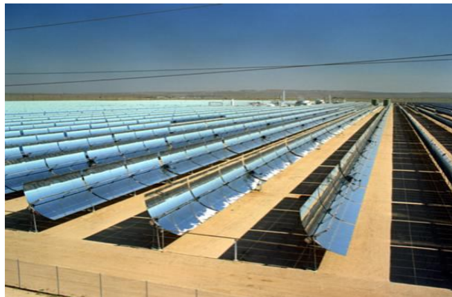
Figure (2.4)Parabolic Trough System.
