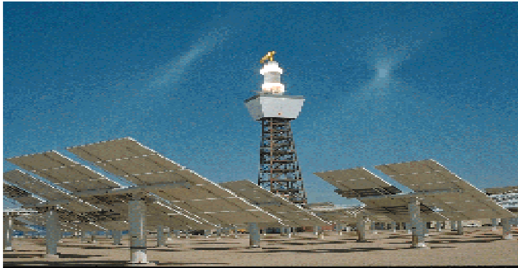
Figure (2.13) Power Tower System With Heliostats.
