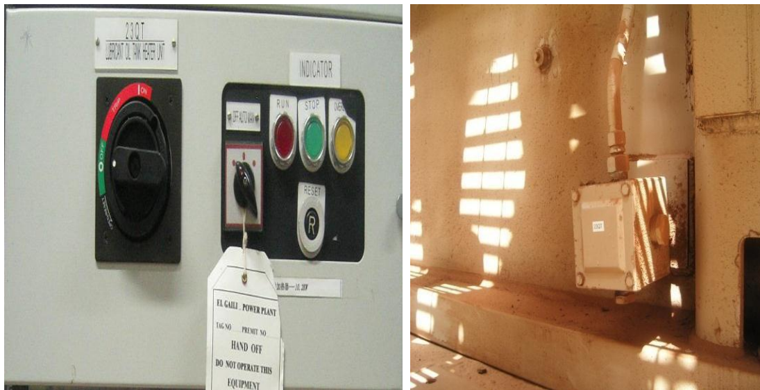
Figure 1 Lube oil heaters
