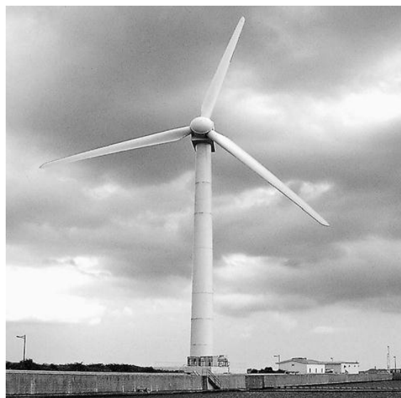
Figure 2.6: 3-blade HAWT,2MW,Okinawa,New Energy Development Company-(Japan).
