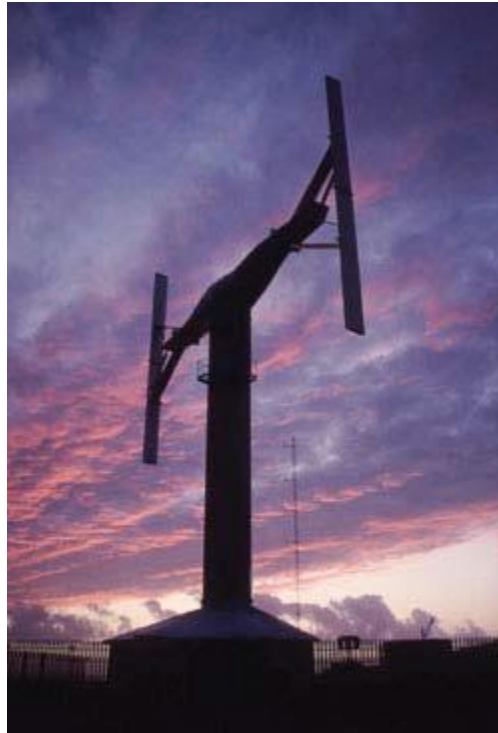
Figure 2.3: A H- type VAWT built in Wales, rated power 130 Kw
