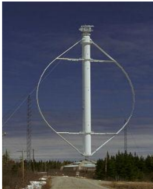
Figure 2.2: A 4 MW, Darrieus-type VAWT, Cap Chat, Quebec, late 1990s.
