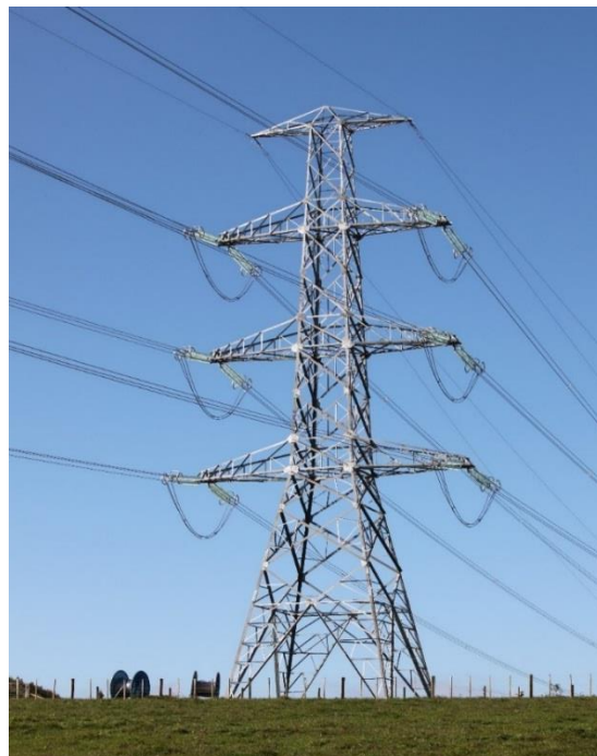
Figure 2.8: Dead end tower.
