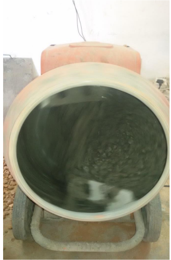
Appendix (E.2): Mixing of concrete components
