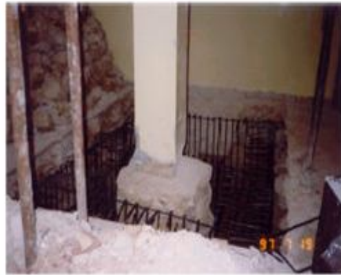
hardening the surface and installing the dowels.
