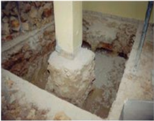
Excavating around the footing.
