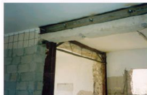
Strengthening by steel plates.
