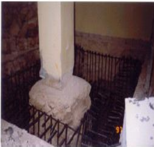
Installing the main steel.
