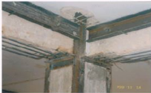
Strengthening a beam , slab and column.
