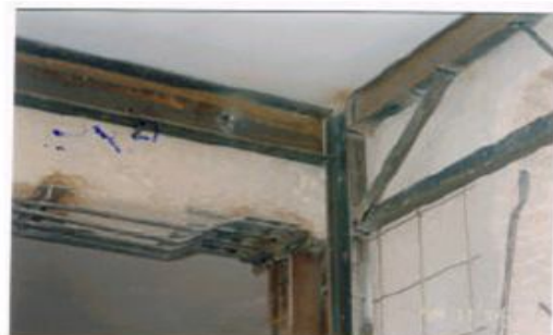
.Strengthening a beam and Slab.
