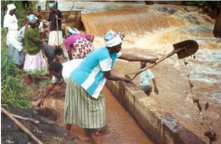
Fig 5. Clearing the canal for Pico hydro power generation (Photo from Martin Wright/Ashden Awards, 2004)
