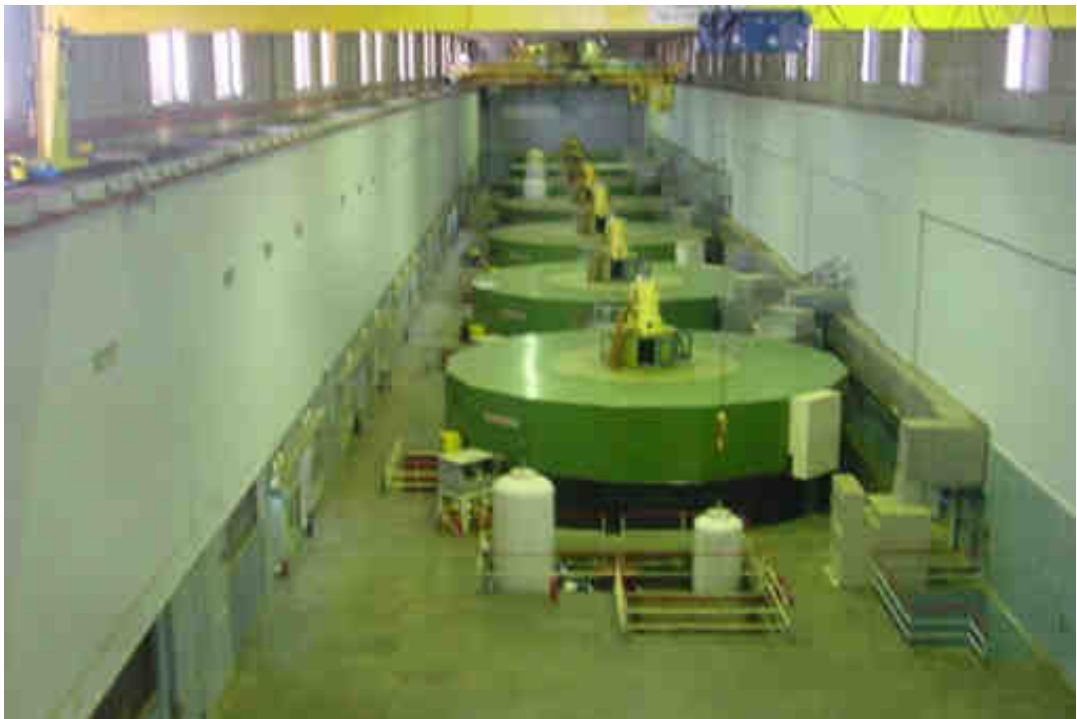
Figure 1.1: 7 Generation units in Rosiers Hydropower Plant
