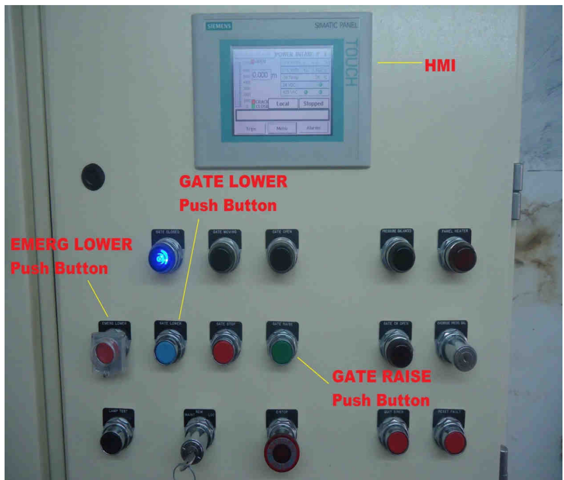
Figure 2.6: Local Control Panel
