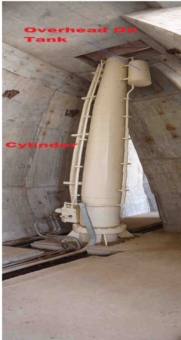
Figure 2.23: Double Acting Cylinder and overhead oil tank
