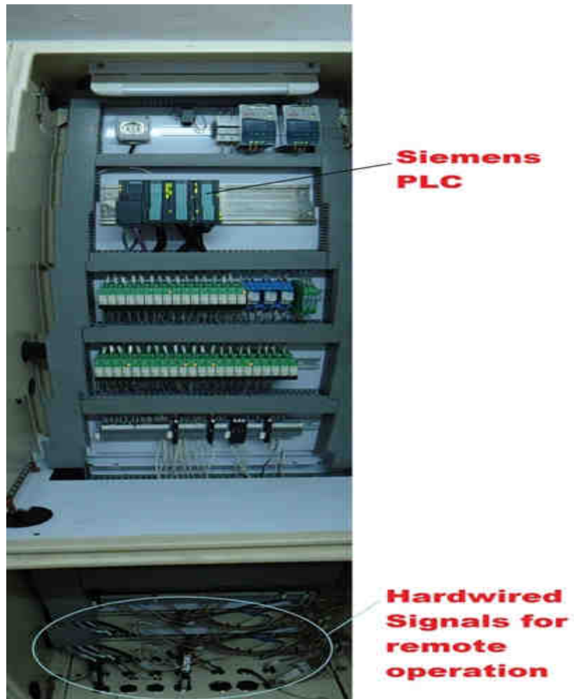
Figure 2.7: Inside Local Control Panel
