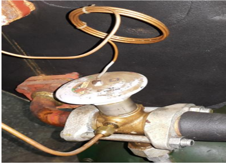
Figure 3-7 Thermostatic expansion devices.
