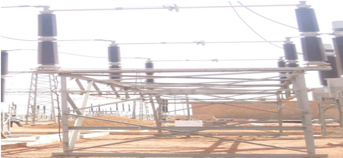
Figure 3.6: The Isolator Swit
