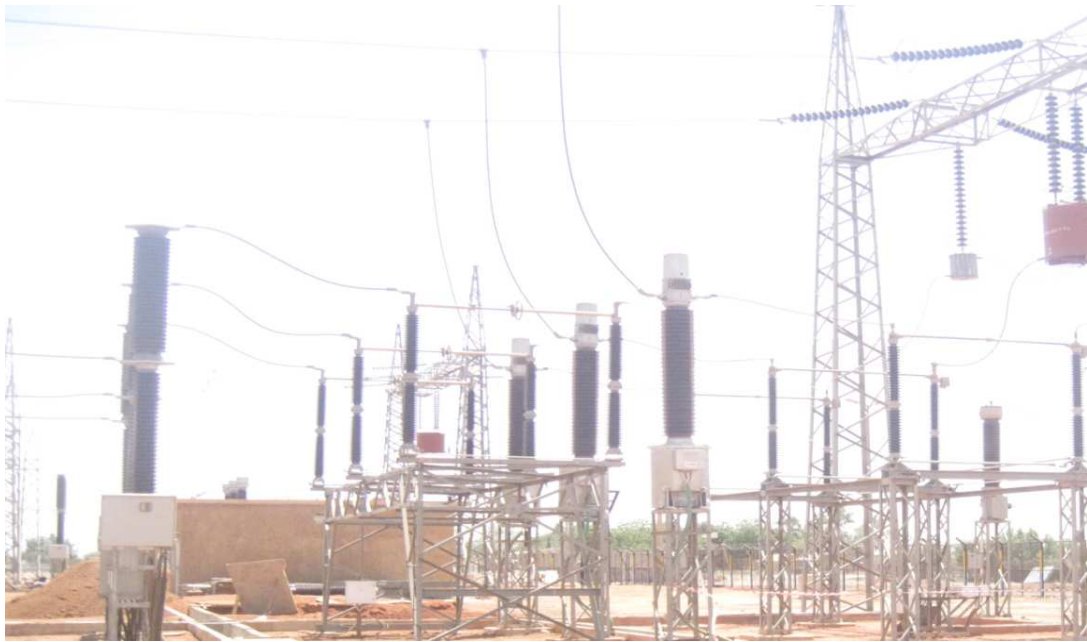
Figure 3.7: the Bus bars Arrangement
