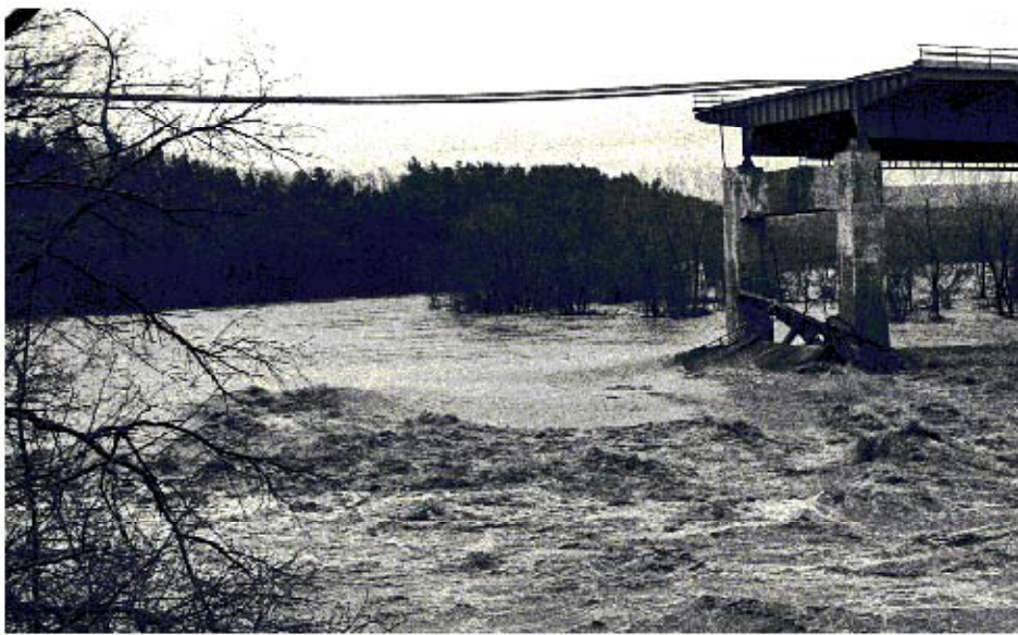
Figure2.2.5 show the accidents due to weather in Schoharie Creek Bridge(Andrzej S. Nowak) (6)
