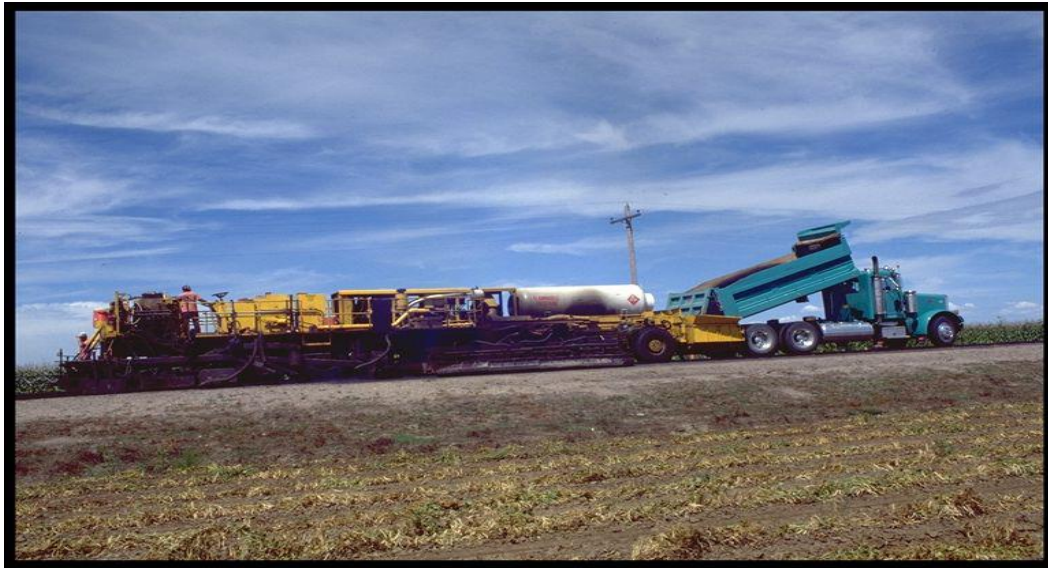
Figure 3-8: Hot in-place Recycling Operation with Application of Overlay (Repaving).
