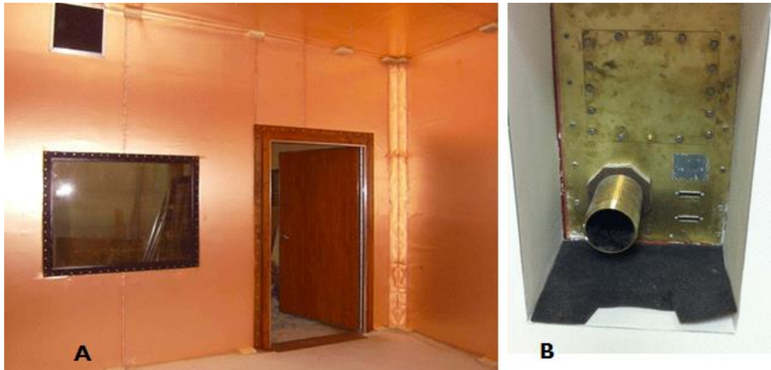
Figure (4.23) MRI shielding, (A) Copper RF-shielding in a magnet room, (B) Penetration panel with protruding waveguide through which hoses and tubes may be passed.
