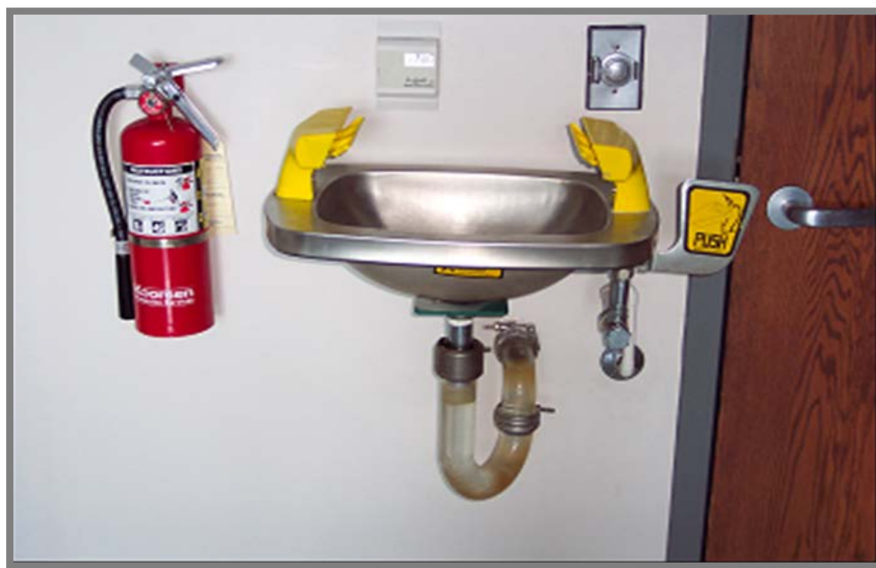
Figure (5.14a) Device use to irrigate and flush both the face and the eyes.
