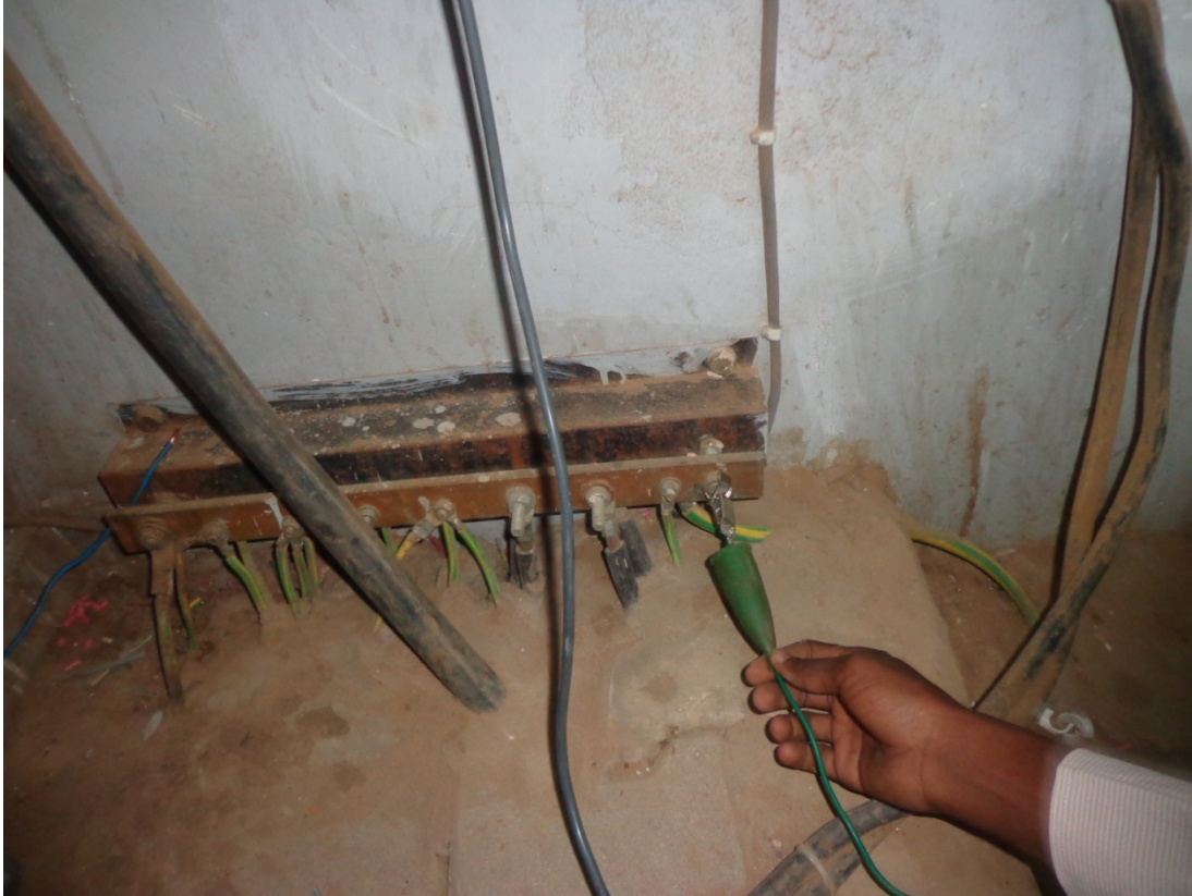
Figure 5.7: the image showed connecting digital earth tester pole (green pole) to the main earthing terminal in case five hospital.
