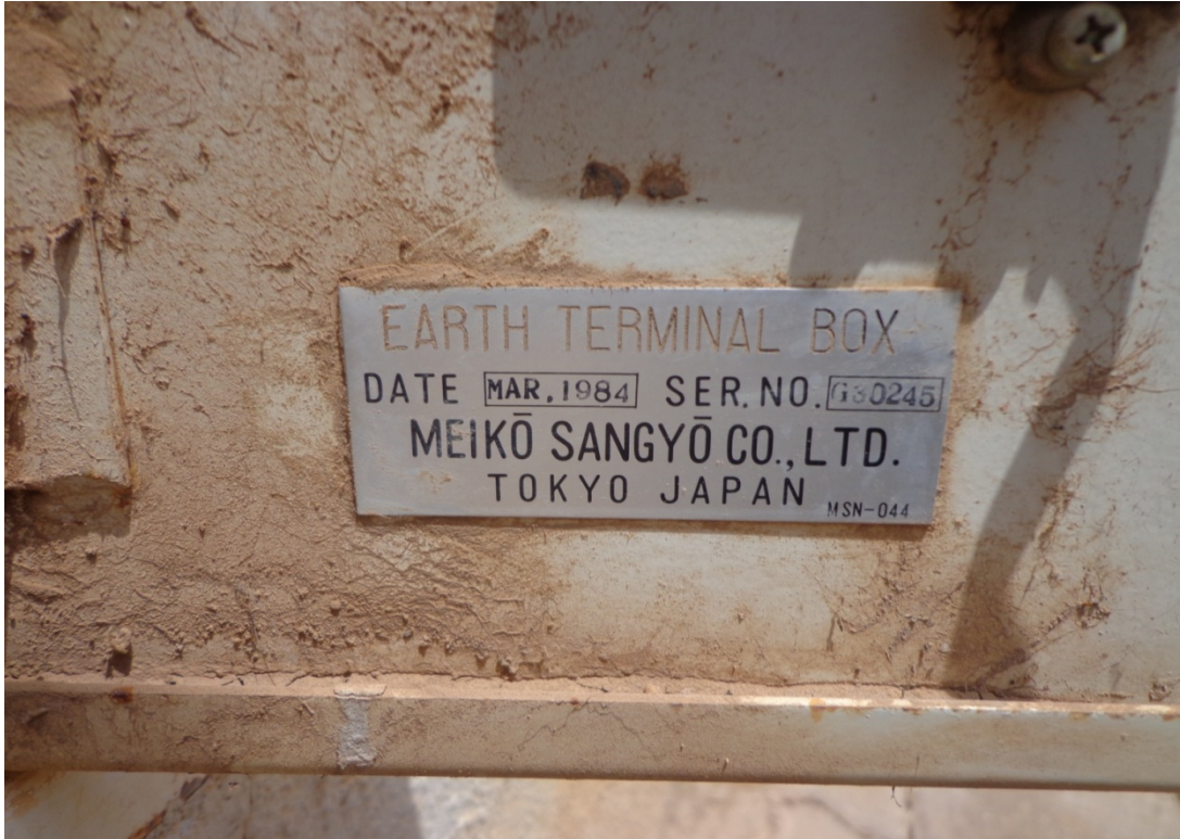
Figure 5.1: image showed the earth terminal box which contains the main grounding terminal in case two hospital captured by researcher camera.
