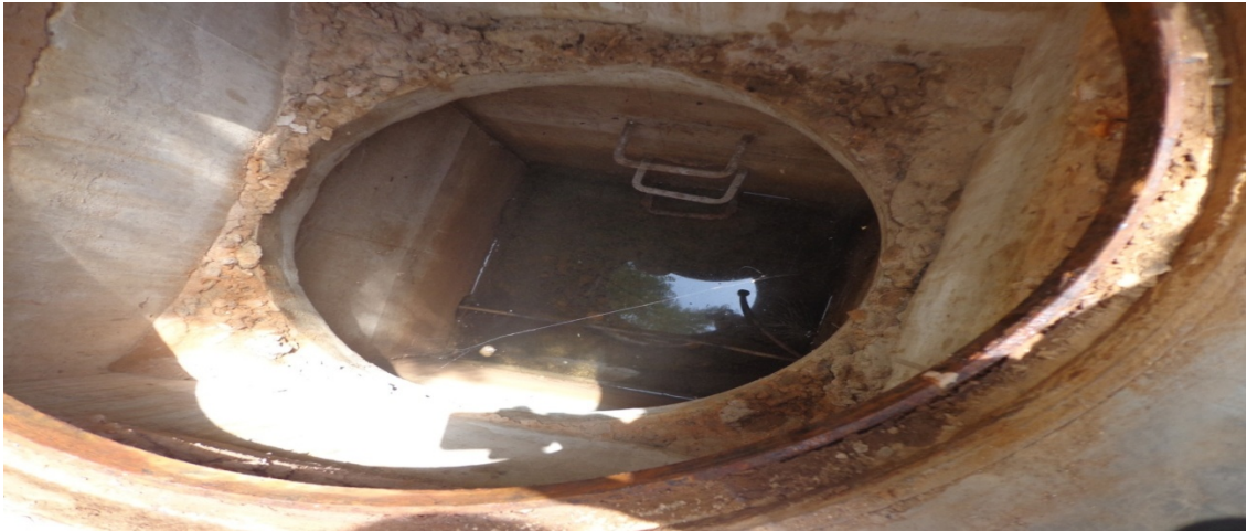
Figure5.2: image showed one of the inspection points of the earthing system which is mixed with the sewage in case two hospital.
