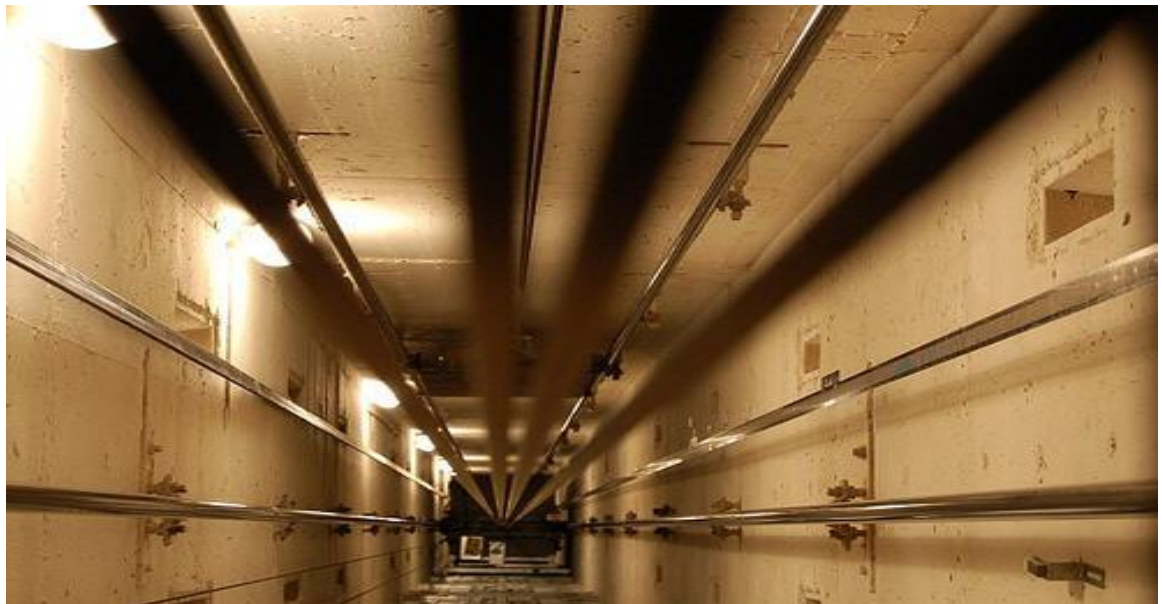
Figure 2.4 Hoistway.
