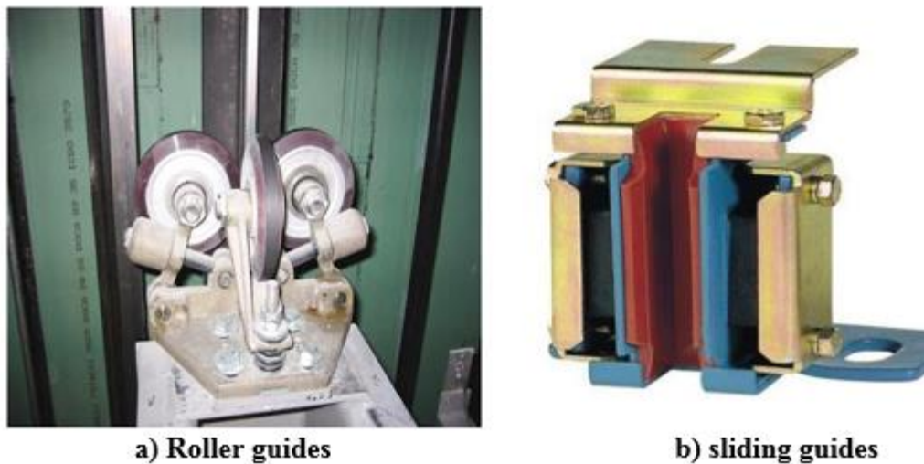
Figure 2.5 a) roller guides b) sliding guides
