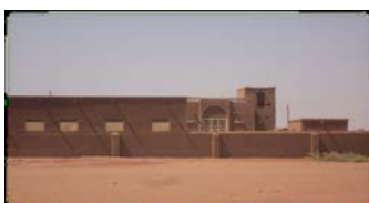
A building in a medium state
