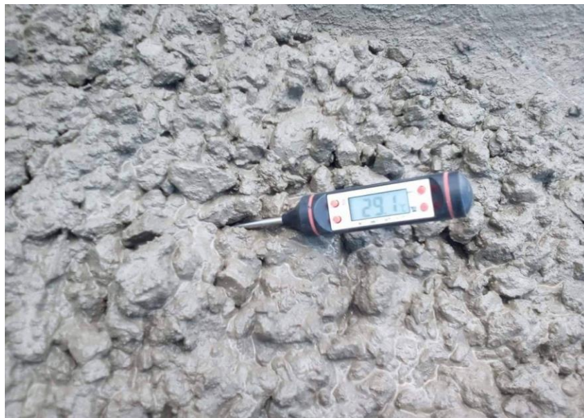
Figure 3.6: Fresh Concrete Temperature Test
