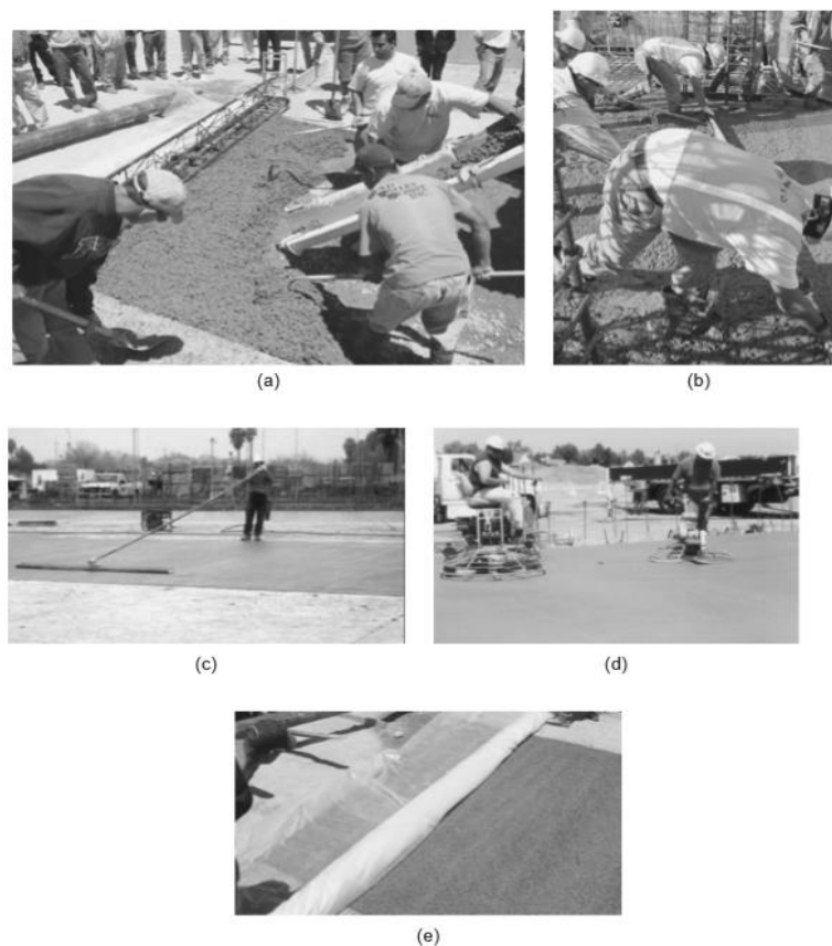
Figure 2.8: Placement and finishing of concrete slabs. [3]
