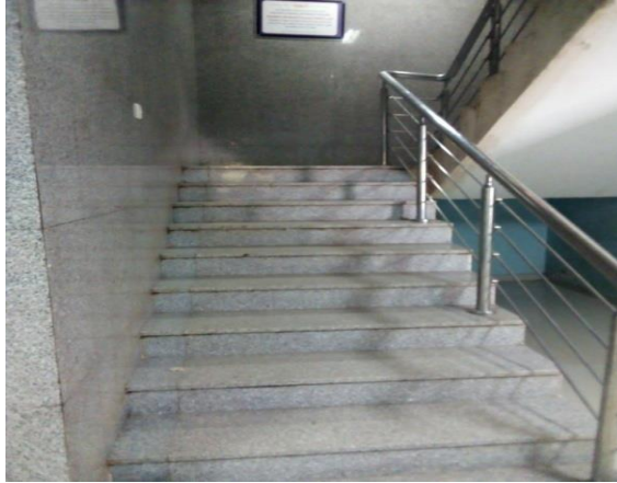
Fig 4-24 Al-moalem hospital's stair Source: (taken by researcher)
