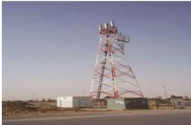
Figure (2.12) An image of Self-supporting towers.
