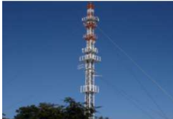
Figure (2.13) an image of a Guyed Tower.
