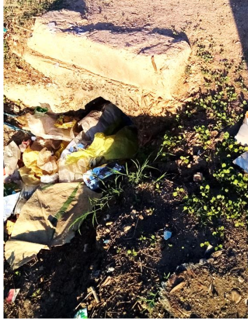
Figure (2.4): plastic bags waste causing blockage of drains.
