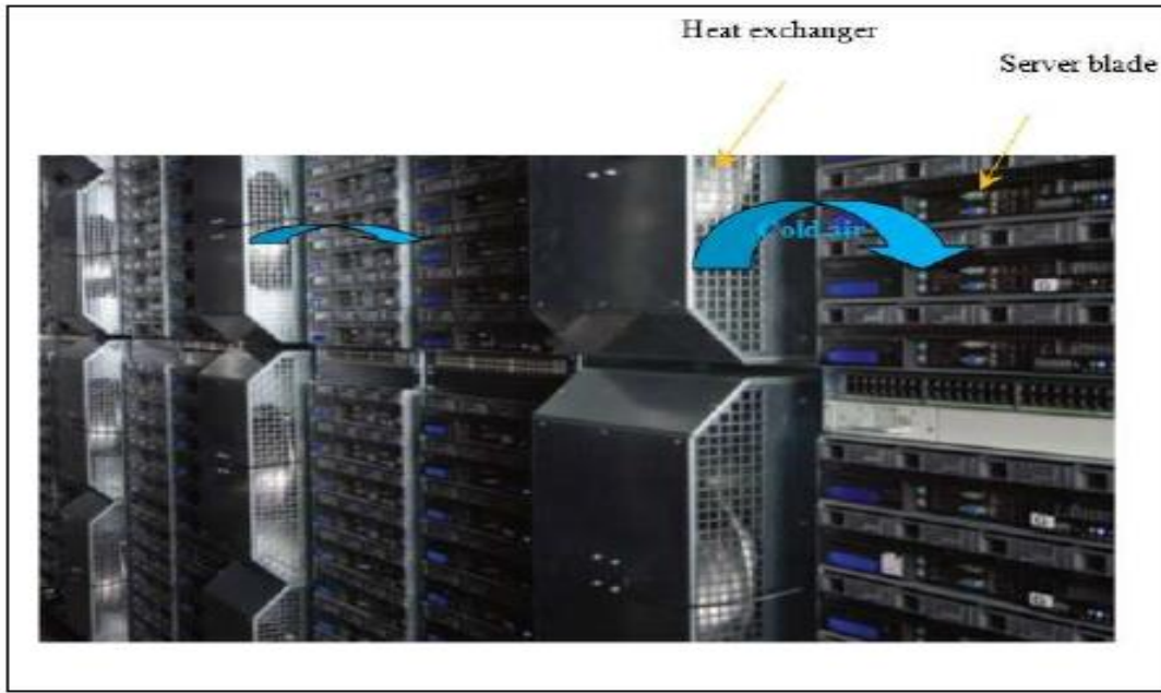
Figure (2-17) Ice cube cooling technique
