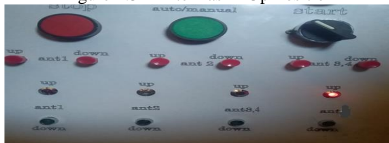
Figure 4.33Indicator of Antennas in Up Position
