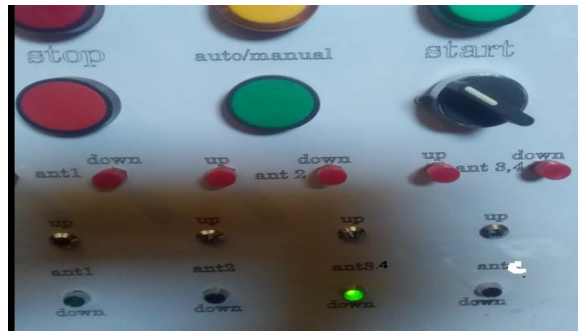
Figure 4.55 Indicator of Antenna 3, 4 Moves to Dawn Position
