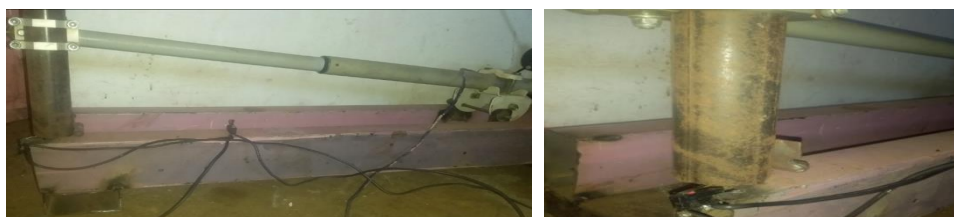
Figure 4.30 Antennas Moves to Up Position
