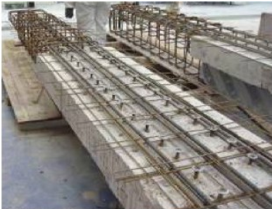
Fig . (4.2 ) Interleaving Between Cantilever and Existing Beam[8R] .
