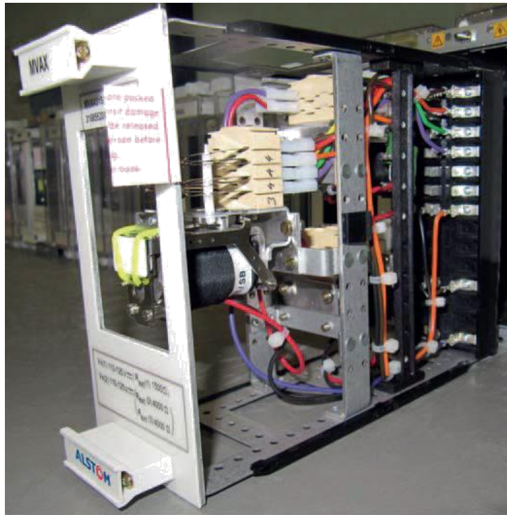
Figure 2.7: Attracted armature relay.
