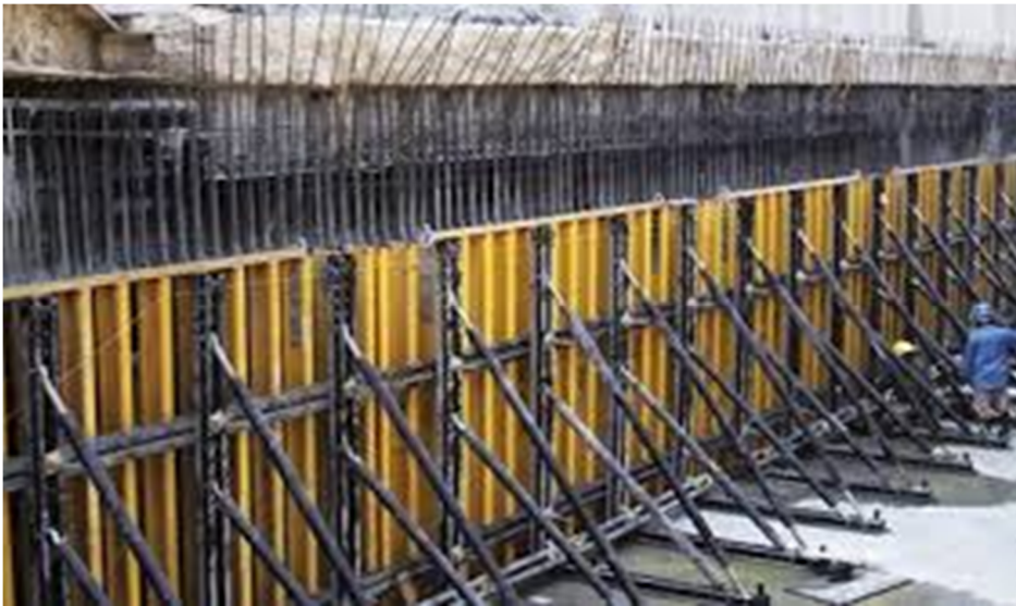
Fig (2.7) Wall Form work
