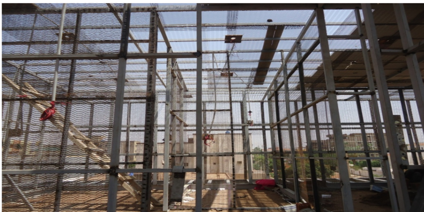
Fig (3.3) light steel framing
