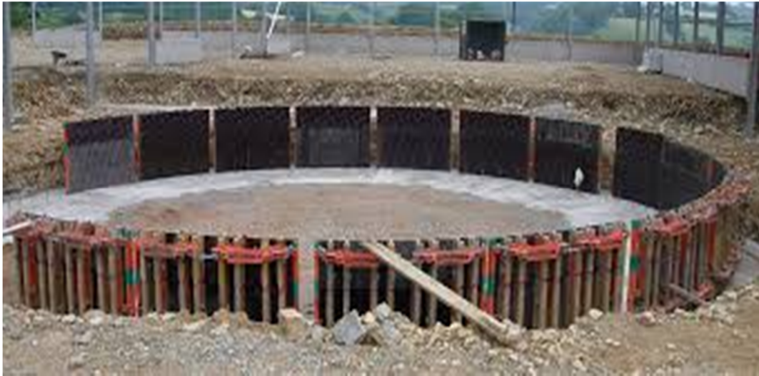
Fig (2.9) Foundation Form work
