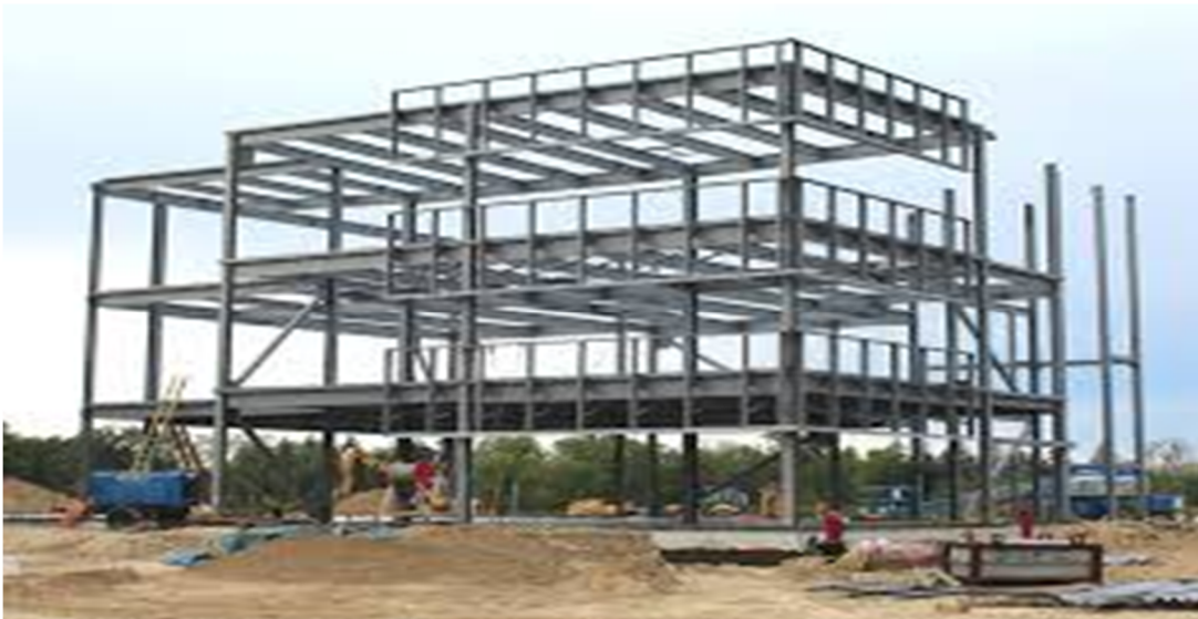
Fig (2.12) Steel framing systems
