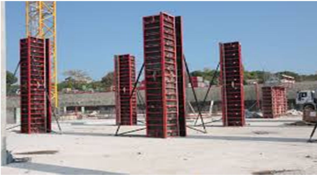
Fig (2.10) Column Formwork
