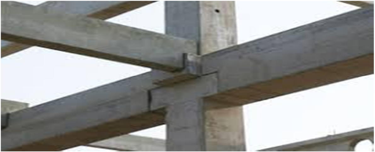
Fig (2.5) Columns and beams
