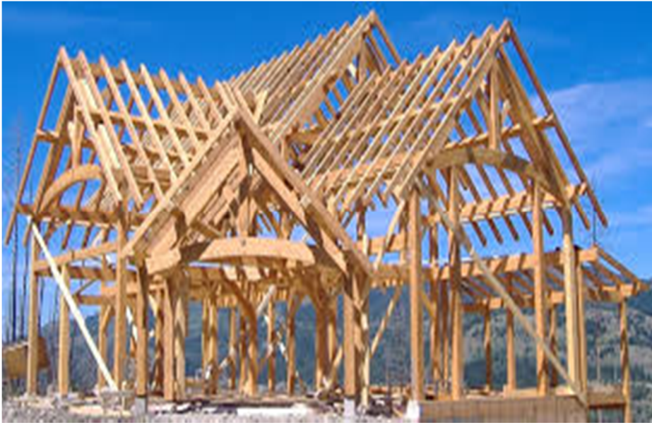
Fig (2.11) Prefabricated timber framing systems
