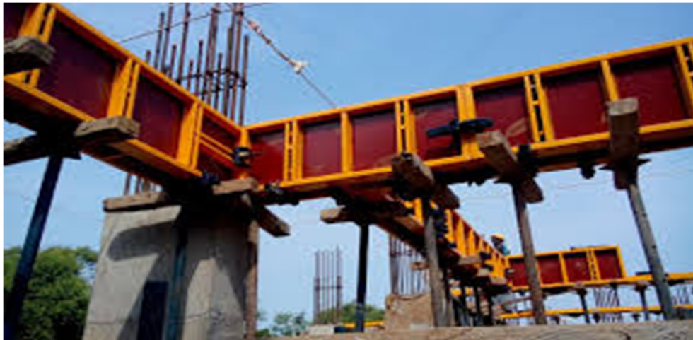
Fig (2.8) Beam Form work
