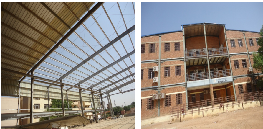
Fig (3.2) steel framing
