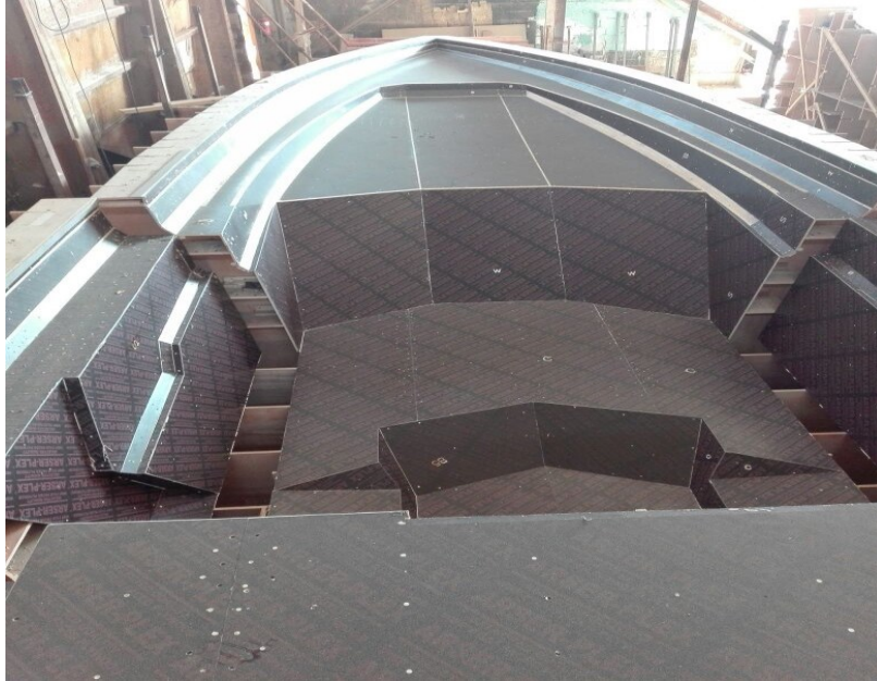
Plywood temporary mold for FIC-15 (SHAMA MARINE -EGYPT)
