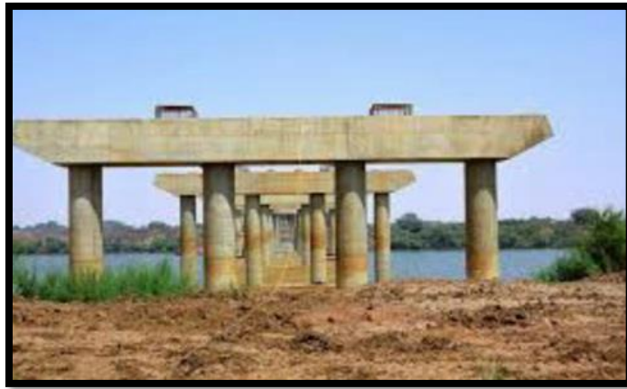
Figure (4.3) Piers bridge
