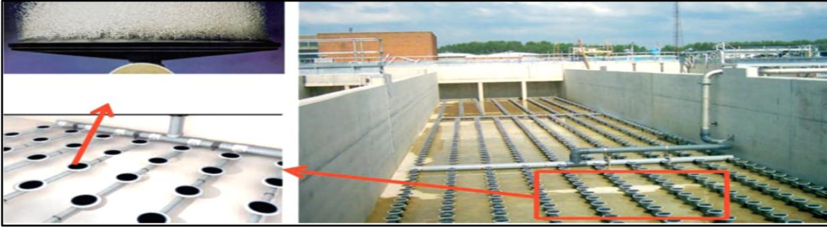
Figure (2-23): Bottom air diffuser grid with one section and fine-bubble dome diffuser [A. Itodo1, 2018].
