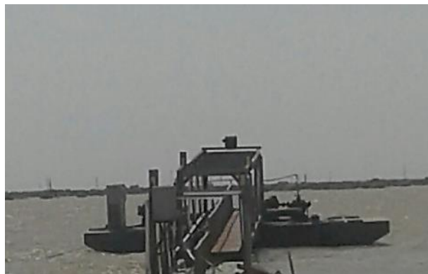
Fig (4.1): Intake at Alshajra Water Treatment Plant
