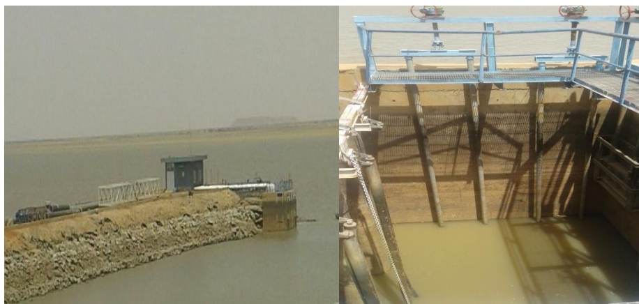
Fig (4.4): Intake at Jabal Awlia Water Treatment Plant
