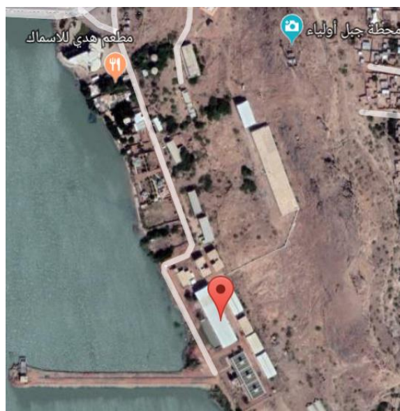
Fig (3.4): Aerial view for Jabal Awlia Water Treatment Plant.
