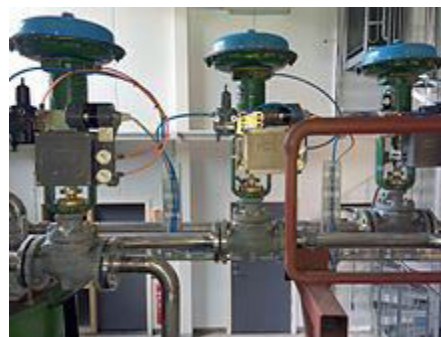
Figure 2. 10 Operation of control valve
