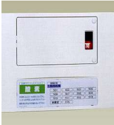
Figures (2-11)-(2-12) Example of Valve: Shut off
