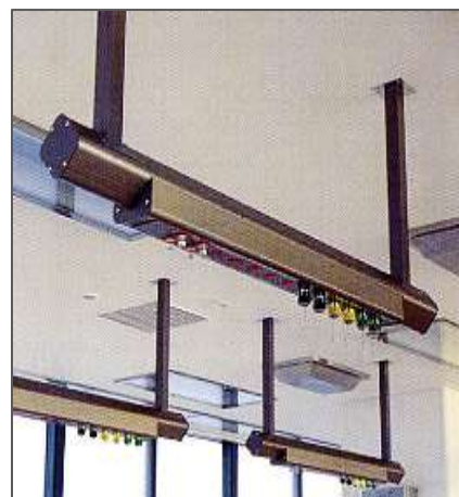
Figure 2-20 Ceiling type Outlet
