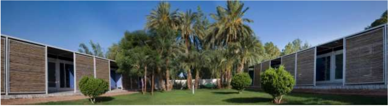
Figure 3-18 Inside Courtyard of the Compound
