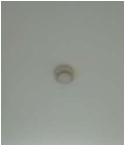
Figure 3-40 Smoke Sensor
