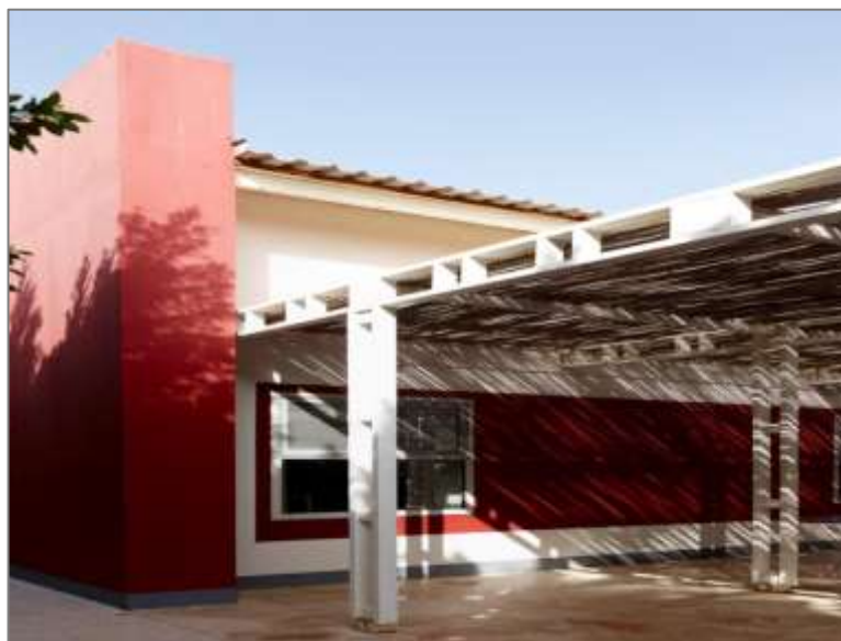
Figure (3-12) Building Views
