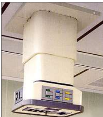
Figure 2-19 Ceiling type Outlet
