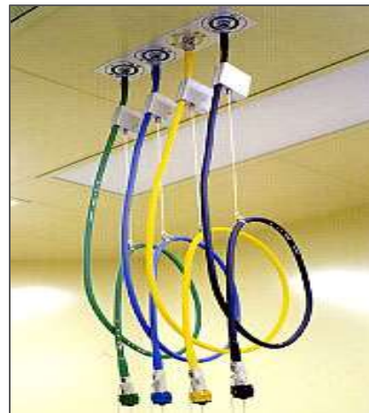
Figure 2-18 Ceiling type Outlet
