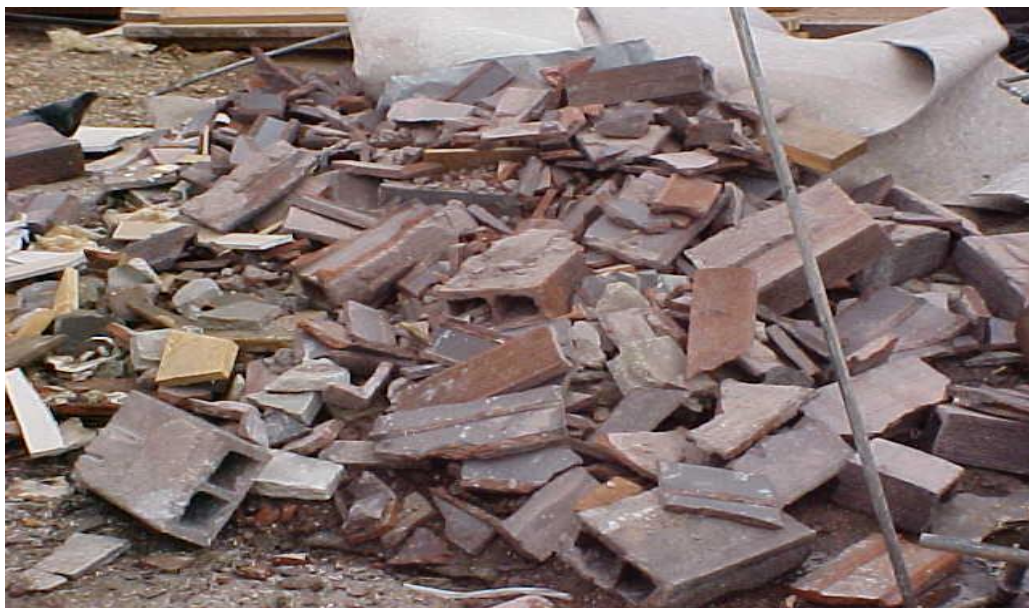
Fig. 2. 2 Bricks/block waste on site
