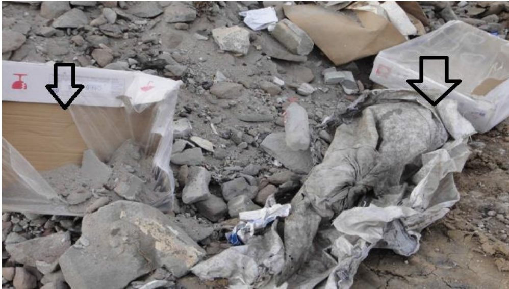
Fig. 2. 5 Papers / bag rubbish on site
