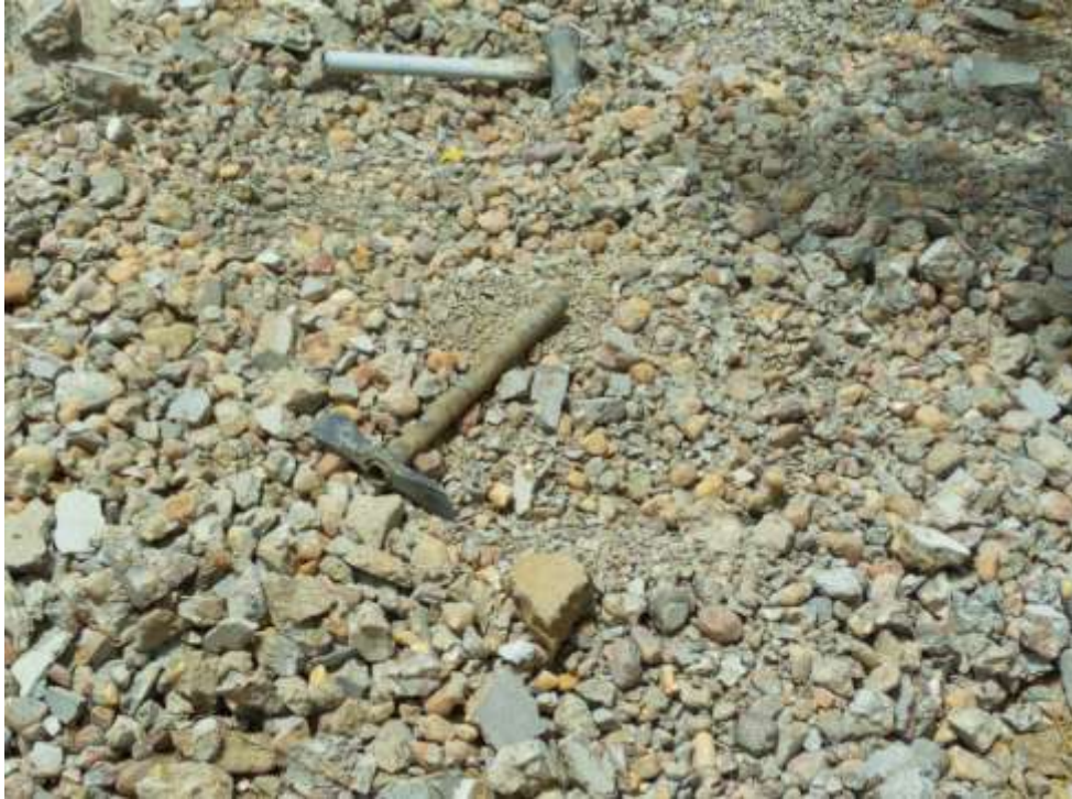
A1 demolition of concrete
