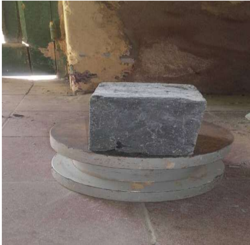
C4 Failure shape
