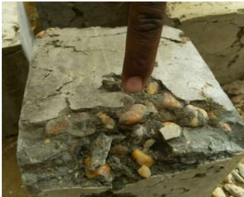
C5 Failure shape
