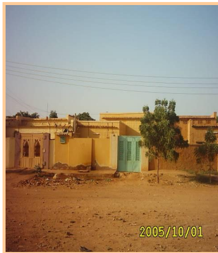
Fig (2-9) low-cost houses In Hai Alomda
