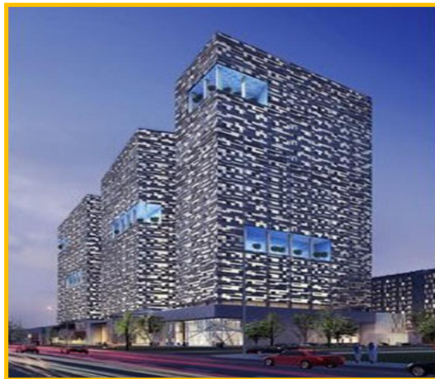
Fig (2-5) Modern Housing Type (Residential complex, Doha). (Source: Tarek Abdelsalam a, Ghada Mohamed Rihaan b, 2012)
