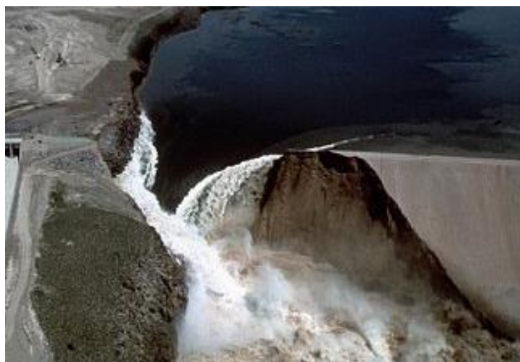
Figure 2-1: Teton Earthen Dam Failure in 1976 (Arthur, 1977).
