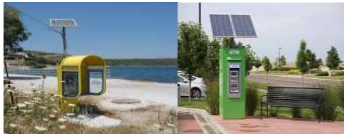
Figure:2.11 ATM and telephone booth powered by PV
