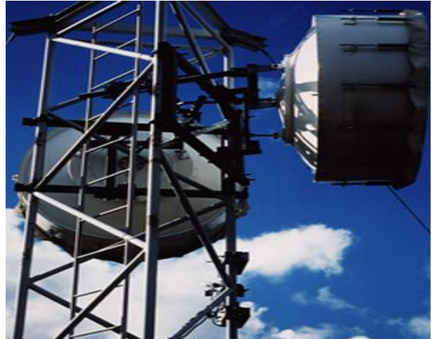
Figure 2.5 Passive relay station (Parabolic reflectors)
