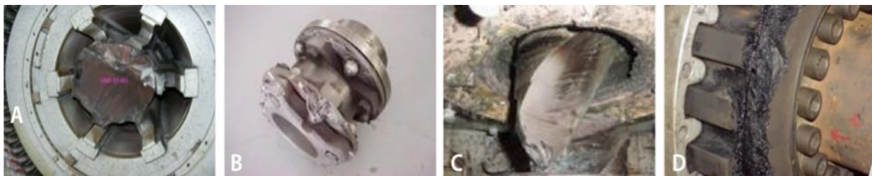
Figure 1-3: sample of failure A) Motor Failure B) Damaged Coupling C) Fractured Shaft D) Melted Rubber Coupling
