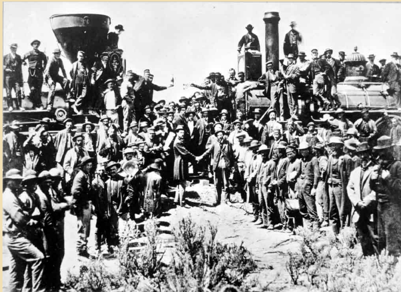
Item 1346 Andrew J. Russell, JOINING THE TRACKS FOR THE FIRST TRANSCONTINENTAL RAILROAD, PROMONTORY, UTAH, TERR. (1869). Courtesy National Archives and Records Administration.
